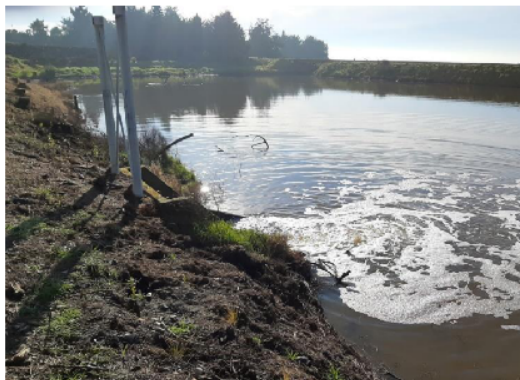
Pumped out flow to Saltwater Creek in operation from the retention pond at Timaru landfill, looking North towards railway bridge over the Creek mouth and Patiti Point.
