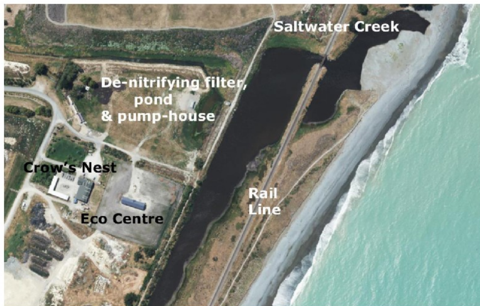
Aerial view of part of landfill site and the Creek north mouth, beyond rail bridge. Also shows stormwater pond and TDC pump house in centre of picture, adjacent to Creek. The edge of Redruth Park is at top of picture.
