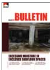
Bulletin 594 Excessive Moisture in Enclosed Subfloor Spaces
