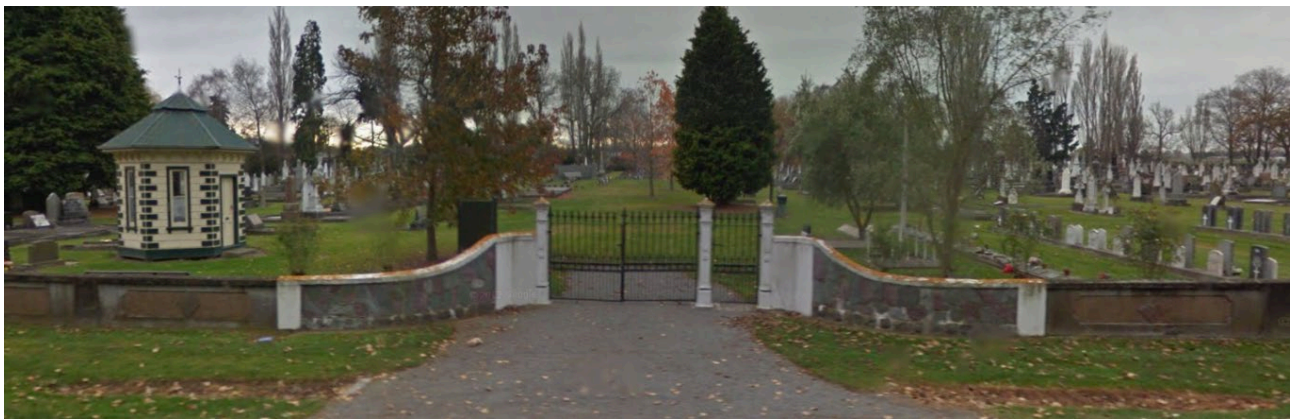
Vestry and entrance gates.
