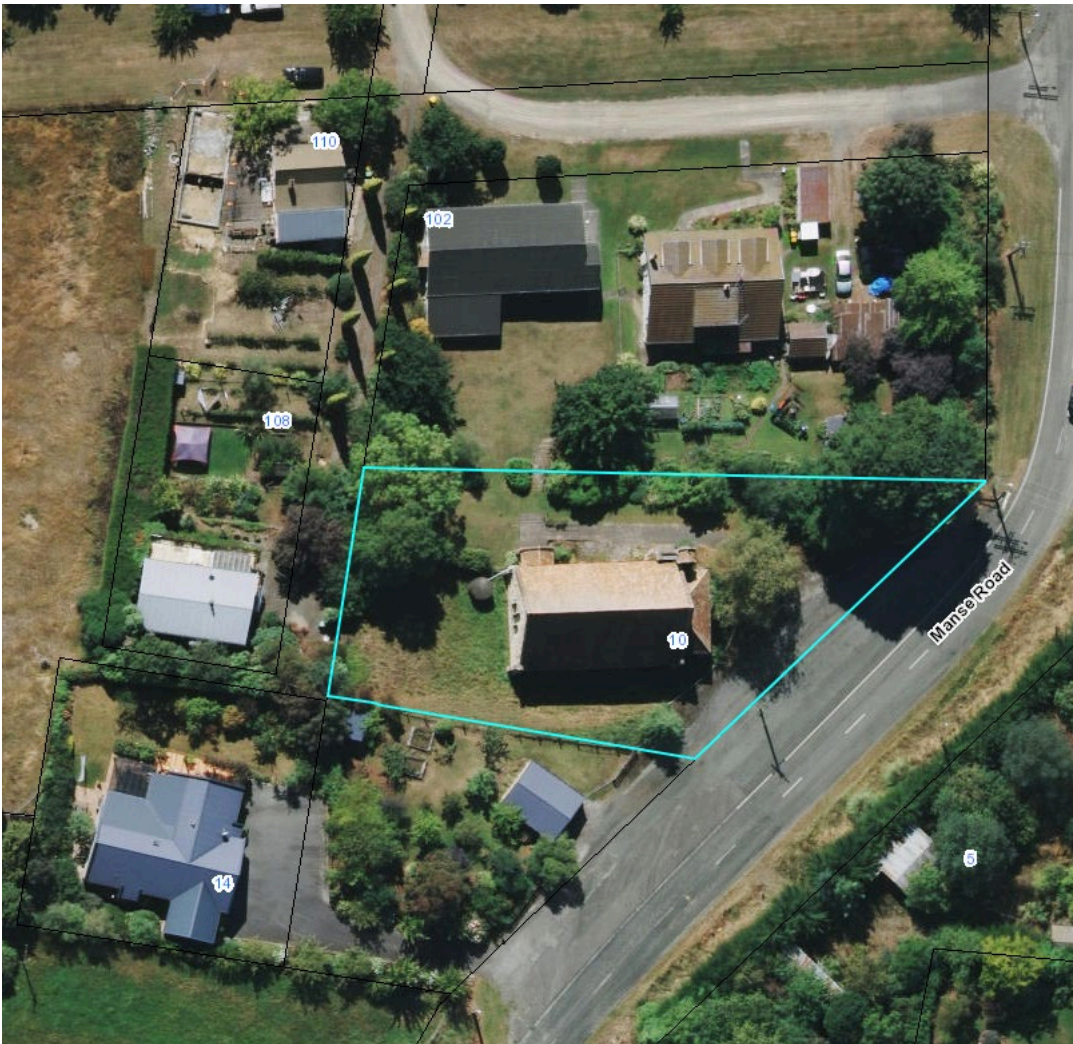
Extent of setting, former St John's Presbyterian Church, 10 Manse Road, Pleasant Point. Church hall and manse are immediately to the north.
