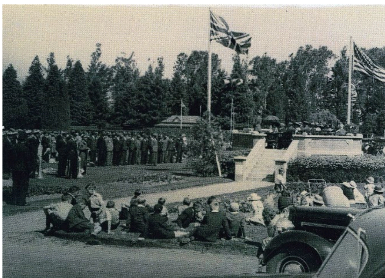
The rotunda accommodating the official party during Governor-General Sir Cyril Newall's visit to Temuka in January 1943. Timaru Herald 26 January 1943, p. 4.
