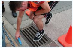
**b.** Remove fish and drill down approximately 40mm
