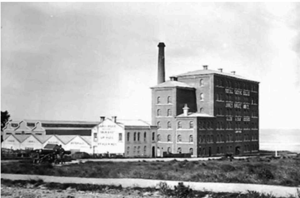
Building before additional two floors added to west elevation. http://diamondmeals.securehost.net.nz/Diamond-History/
