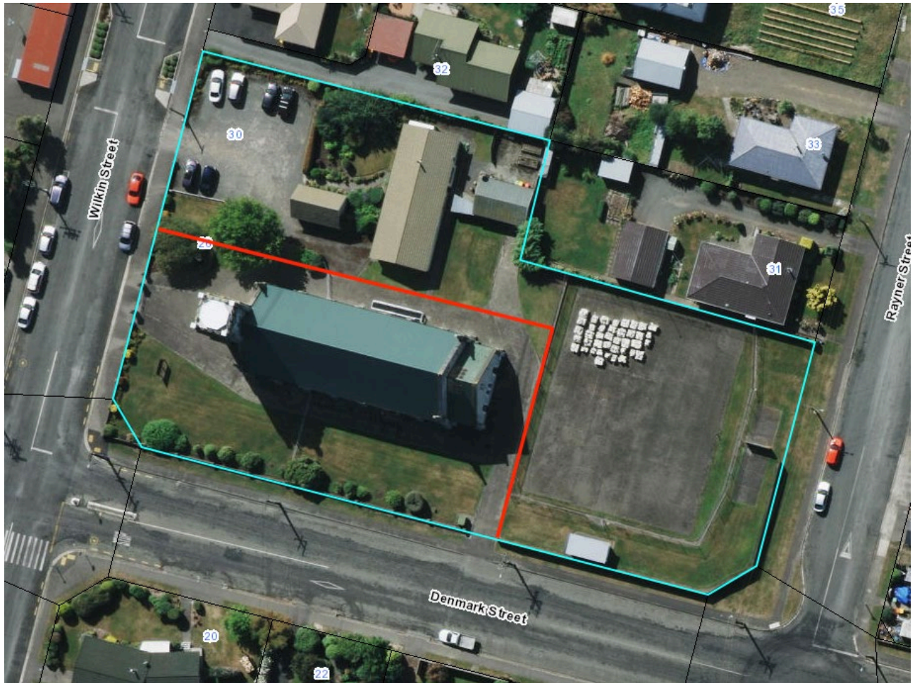
Extent of setting, limited to immediate surrounds of the church, 26 Wilkin Street, Temuka.
