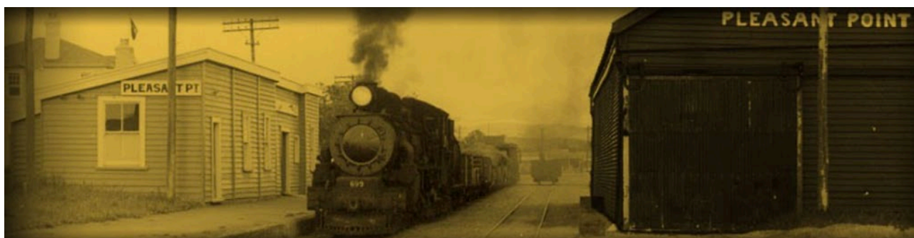
Railway station before canopy was erected and goods shed demolished.
