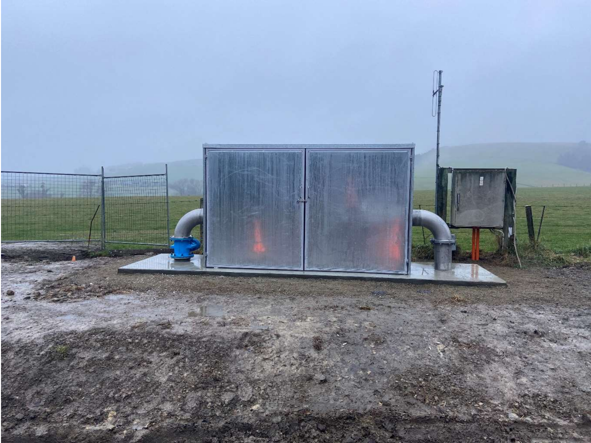
Enclosure in place for Davison Road Water Meter and Strainer
