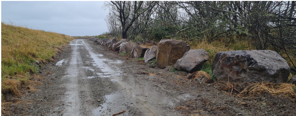
Figure three: Penny Lane in an area that used to be a very deep hole in the track. Newly placed boulders on right. Note that the trees on the right have now been removed.
