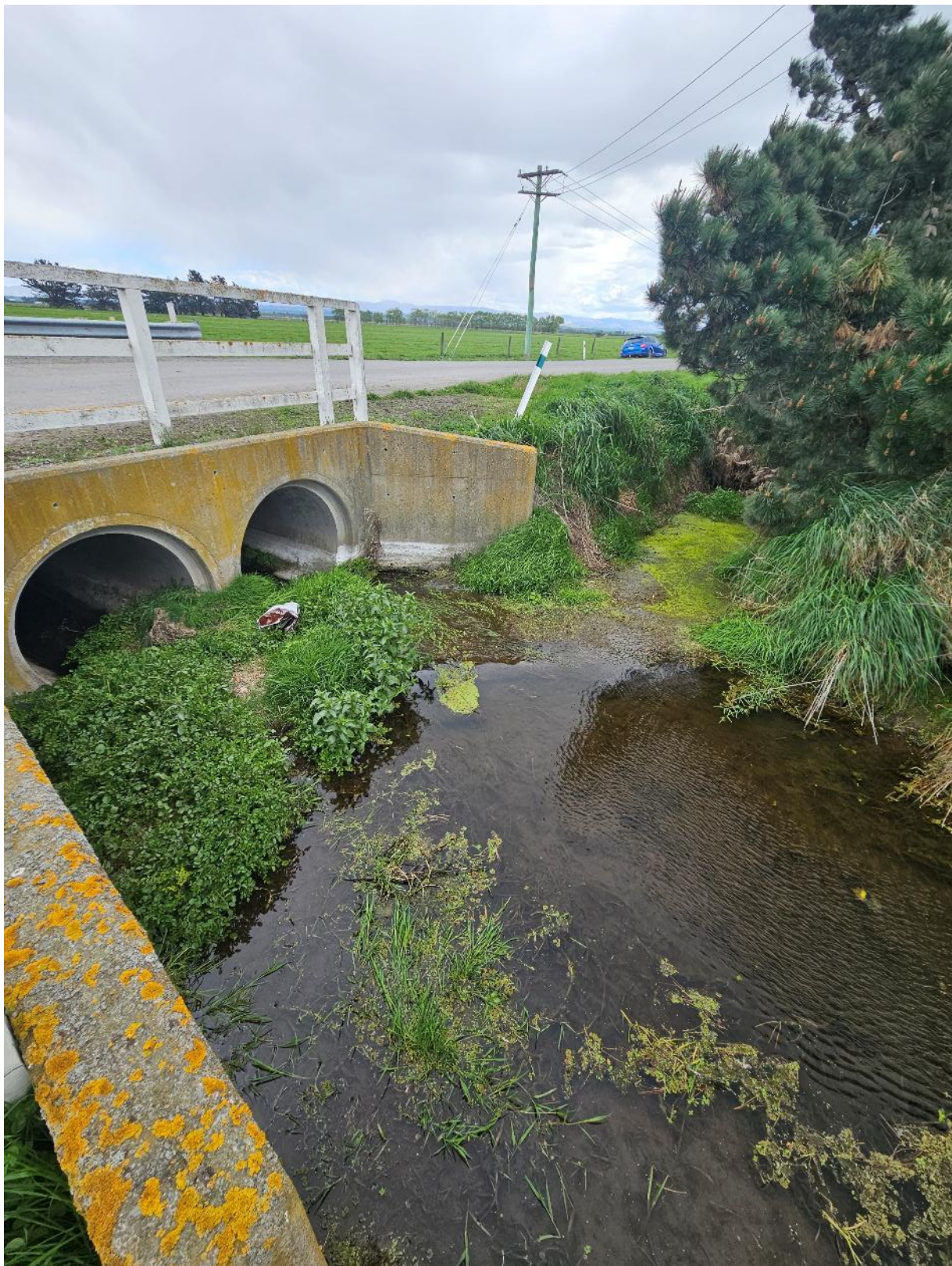
Figure I15: Converging Drains at Corner of Kereta Road and Phar Lap Road (Connecting to Seadown Main Drain)
