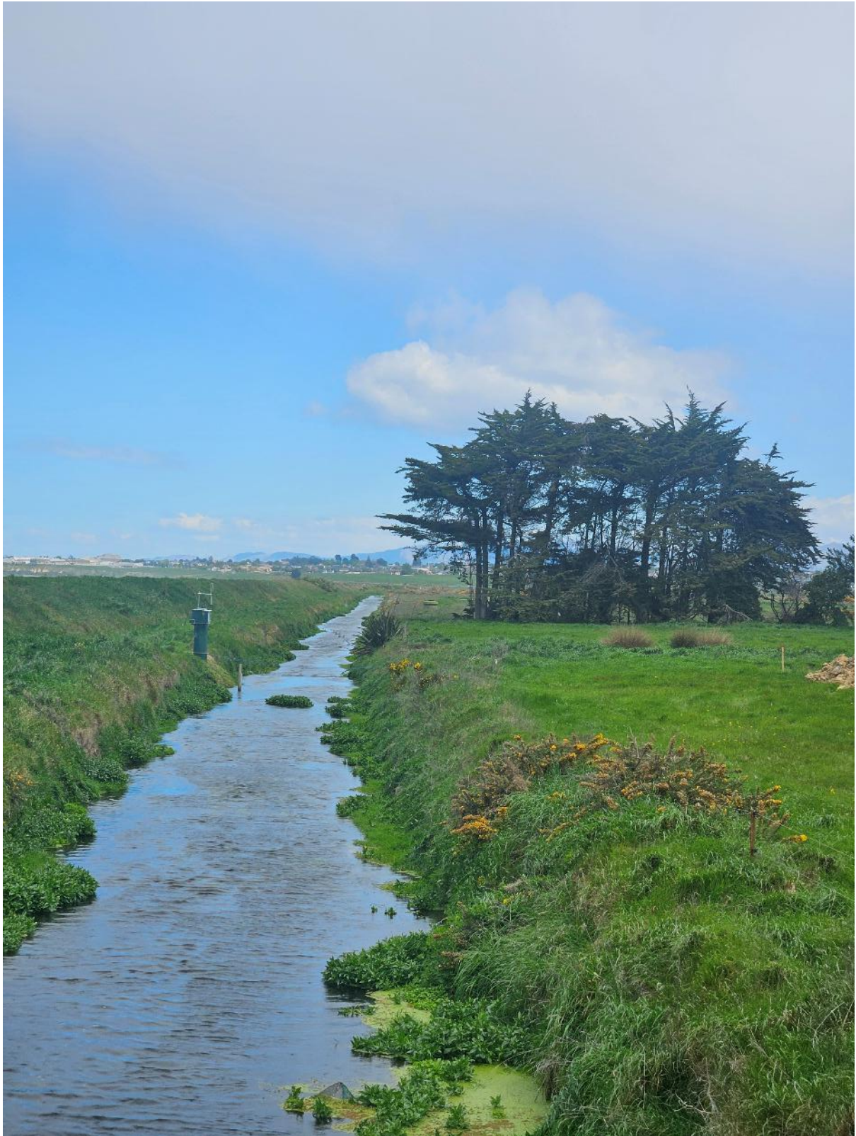
Figure I17: Seadown Main Drain at Aorangi Road (Southward Facing)
