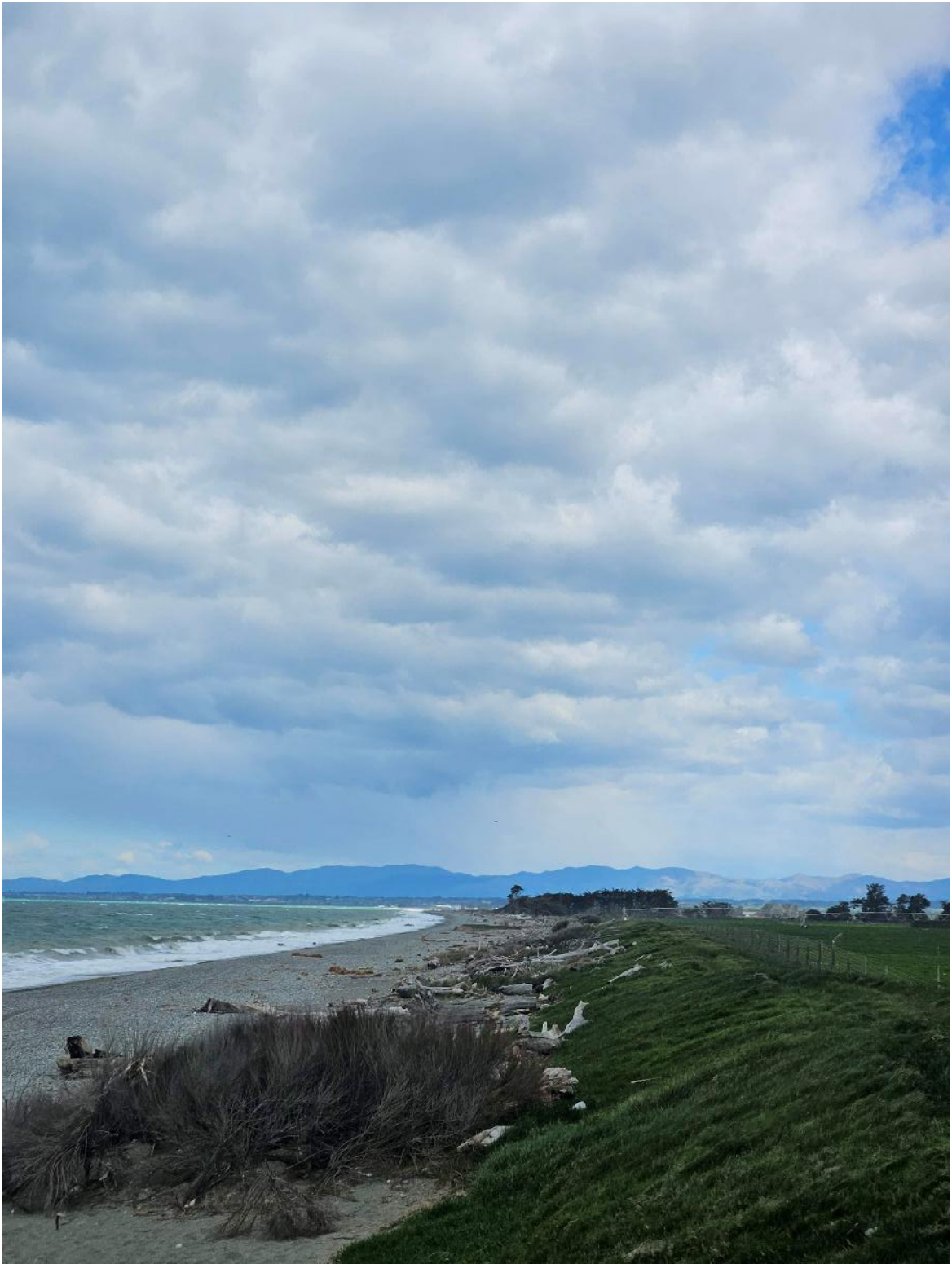
Figure I3: Stopbank at Horseshoe Lagoon (South Facing)
