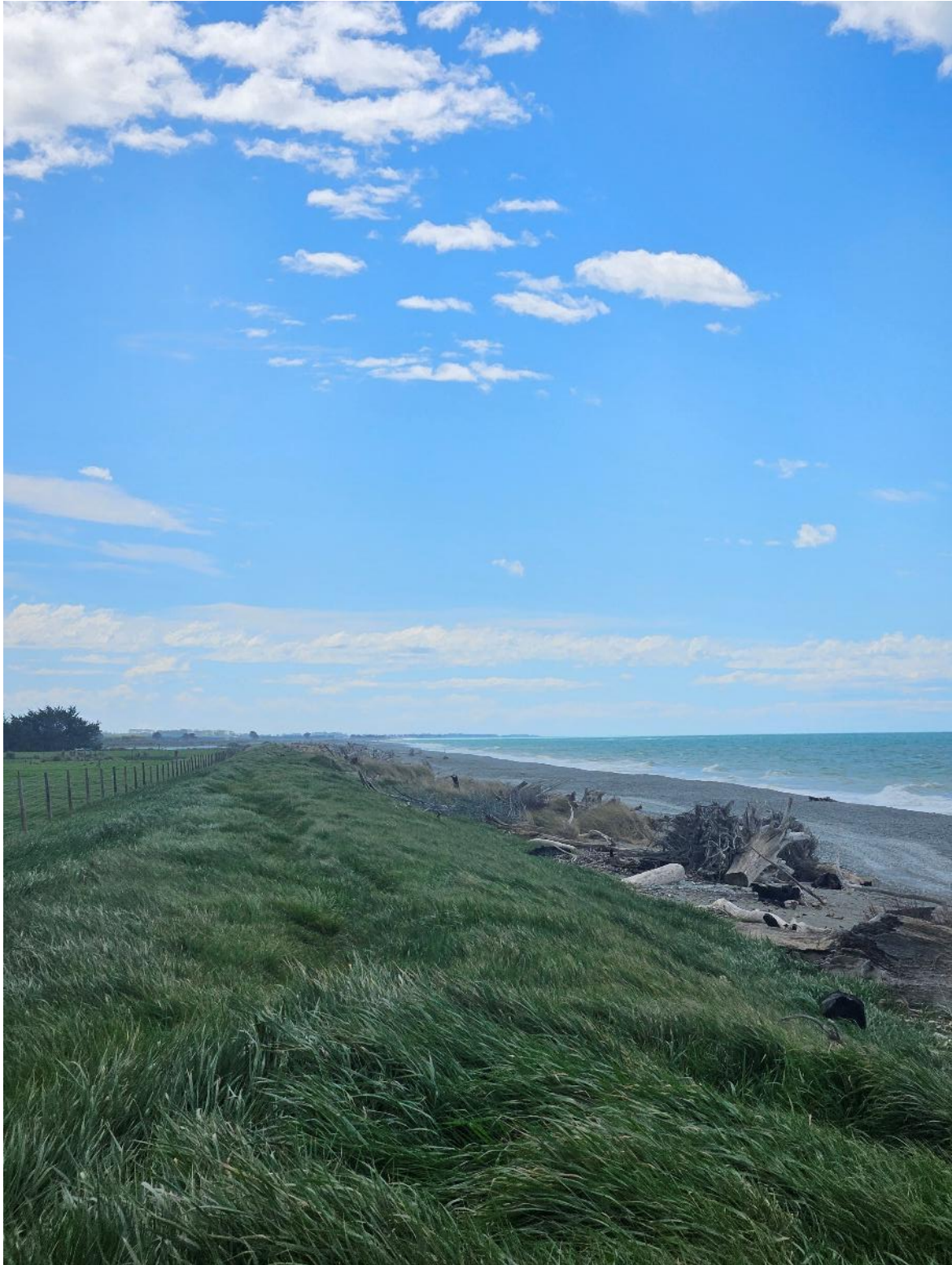
Figure I2: Stopbank at Horseshoe Lagoon (North Facing)
