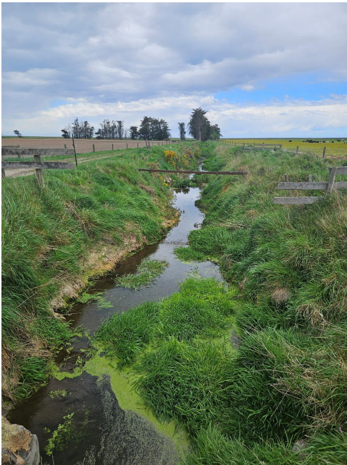
Figure I13: An Additional Drain and Culvert on Kereta Road, Connecting to Seadown Main Drain
