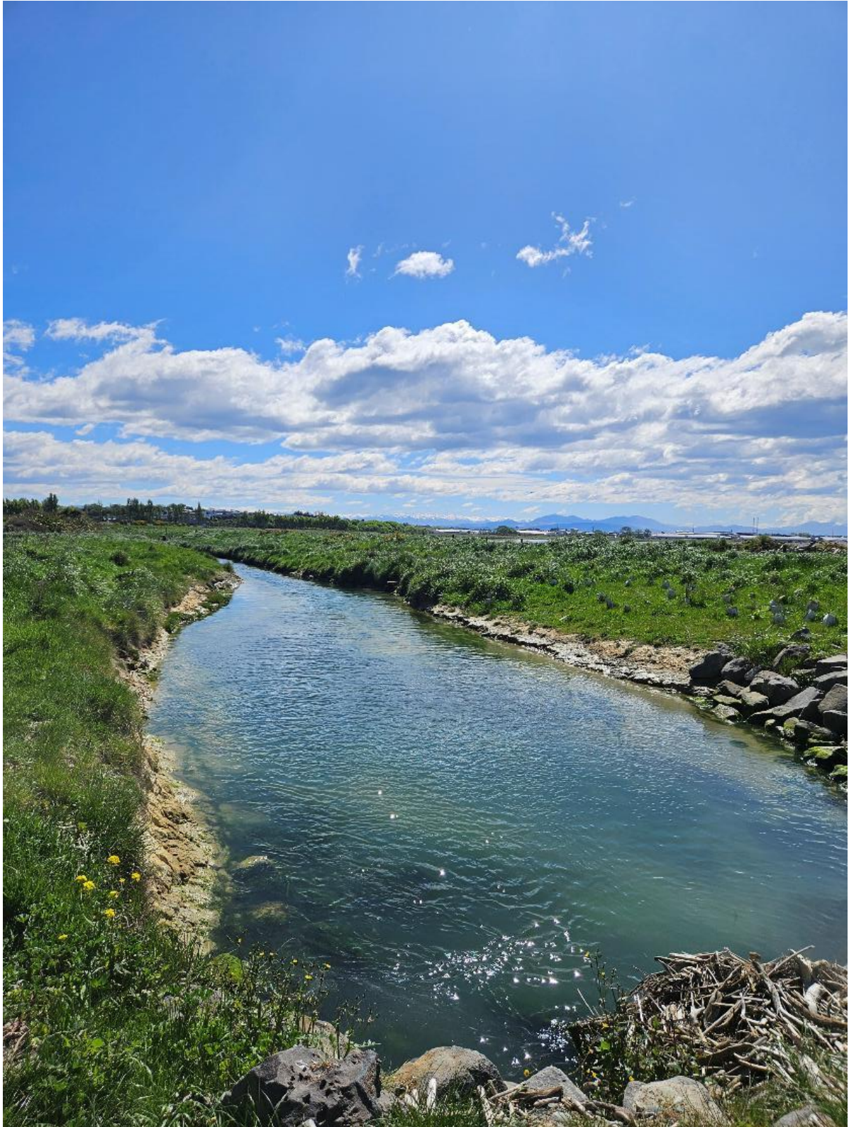
Figure I20: Washdyke Lagoon Ring Drain at Outlet (Facing Westward)
