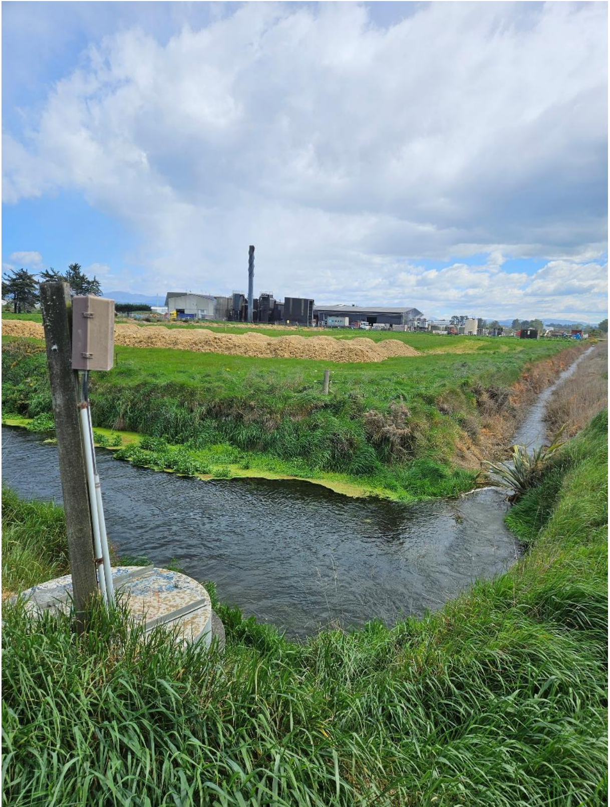
Figure I19: Aorangi Road Drain Entering Seadown Main Drain at Aorangi Road (Eastward Facing)
