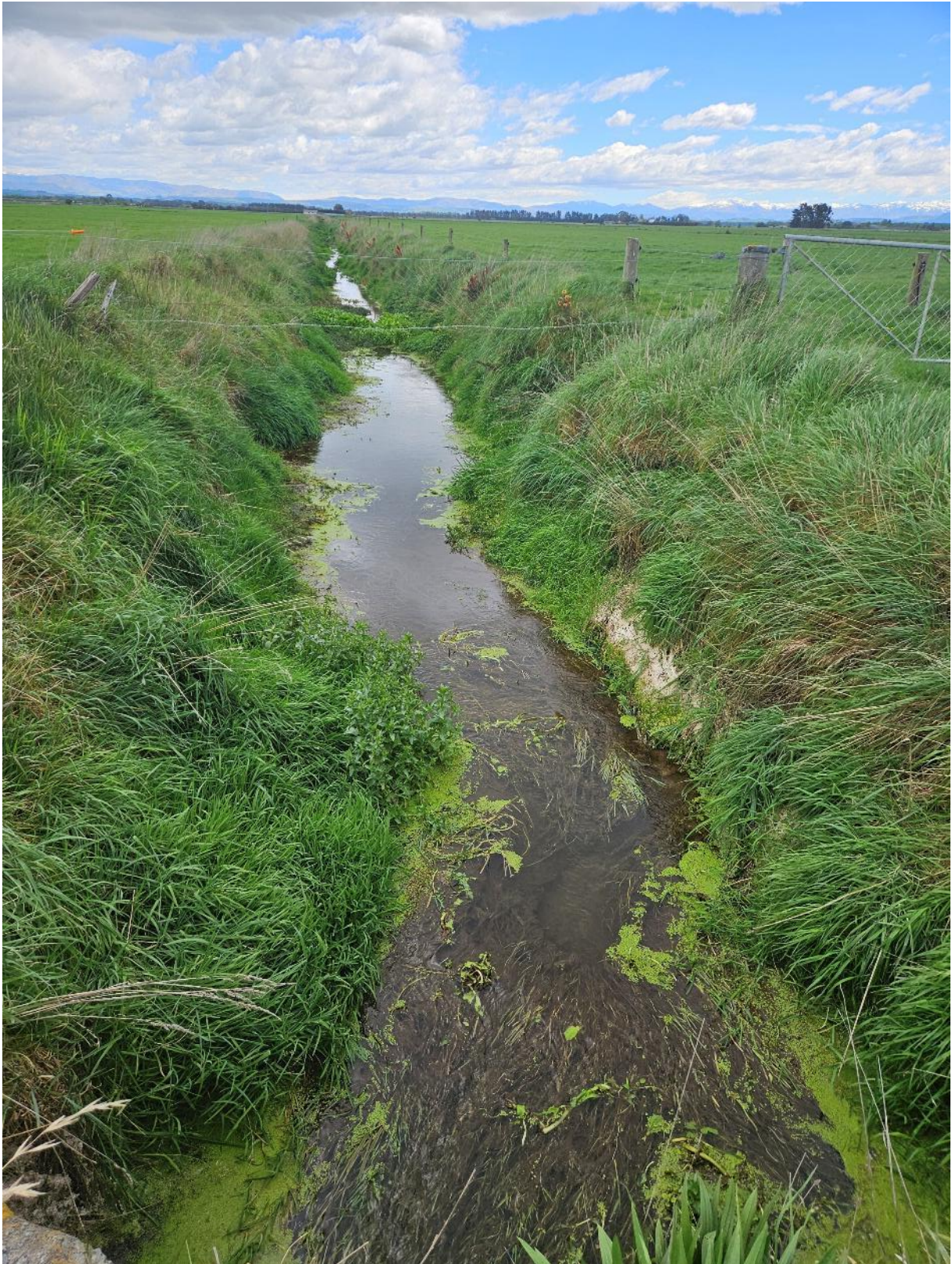
Figure I12: A Drain and Culvert on Kereta Road Drain, Connecting to Seadown Main Drain
