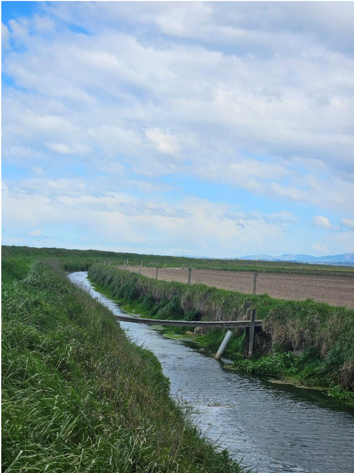
Figure I8: Seadown Main Drain Facing Southward at Philips Lagoon
