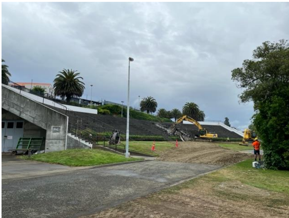
Demolition works, February 2022
