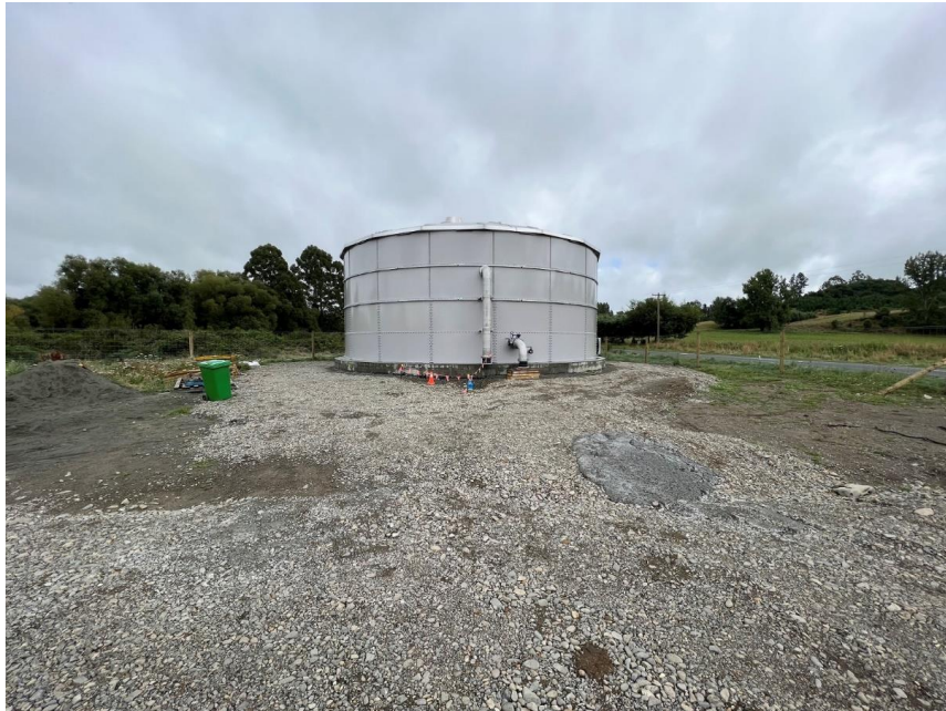
New treated water reservoir (as at 26 January 2022)
