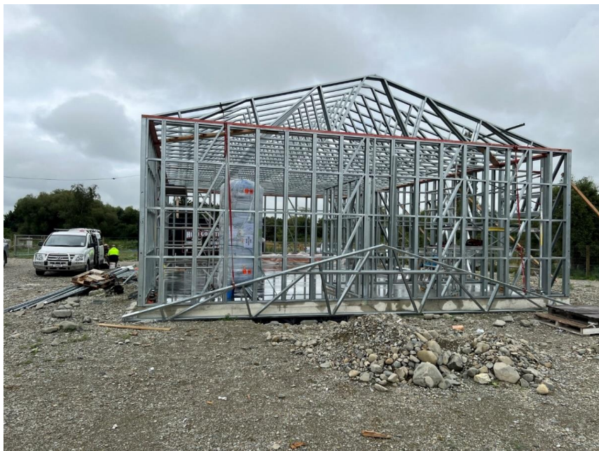
Water treatment plant under construction (as at 26 January 2022)
