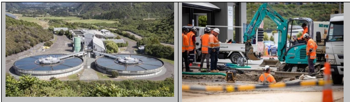
Fig. A3-1 (Left): A Wellington Water fluoridation plant was shut down after an over-dosing incident. Fig. A3-2 (Right): Another challenge for Wellington Water: ageing pipes and associated infrastructure for water, wastewater, and stormwater.
