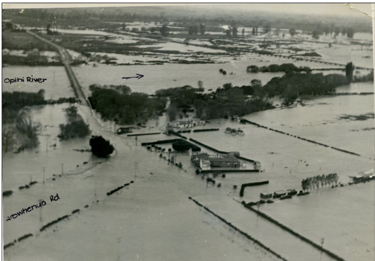
Figure 4-14: 18 April 1951 – flood water flowing across SH1 towards the Waipopo study area
