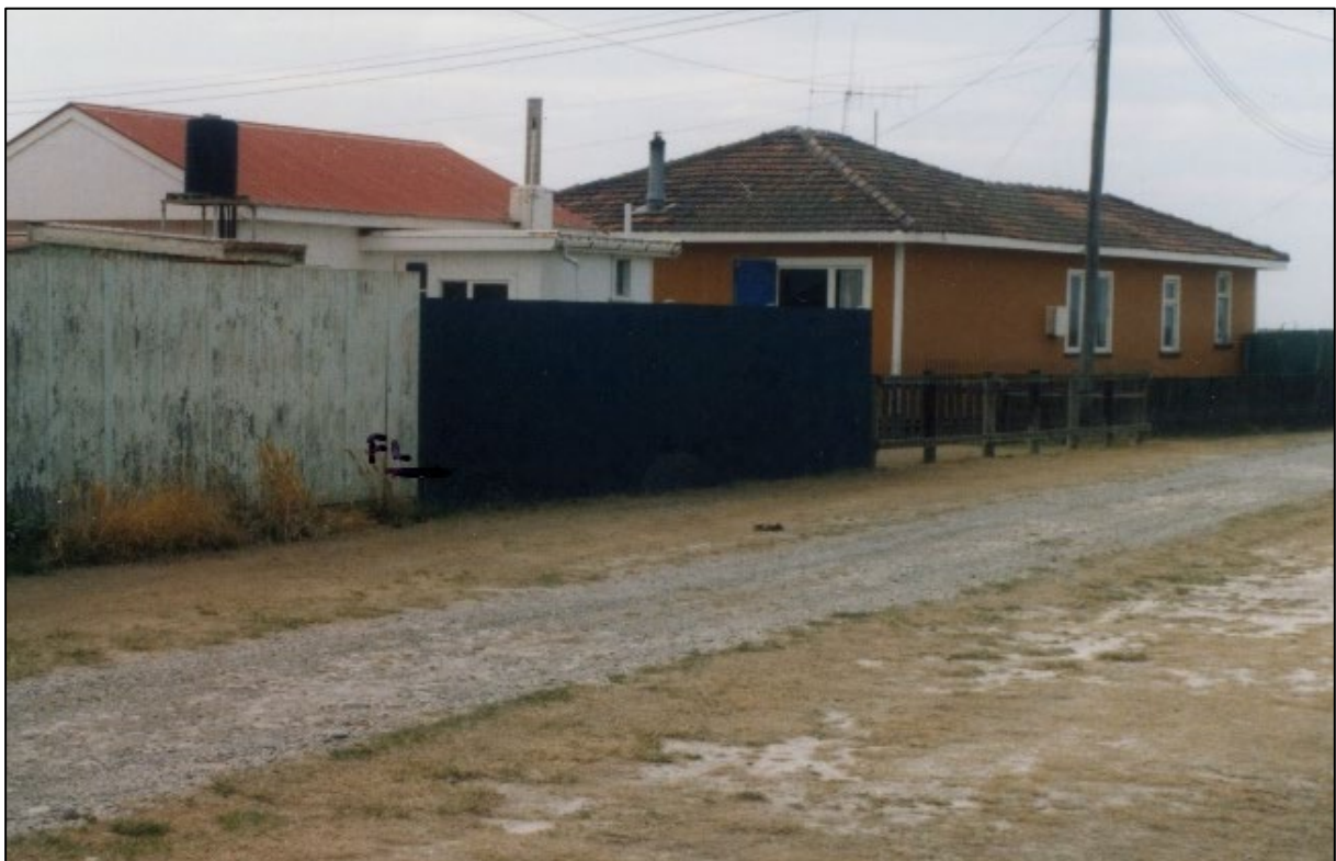
South Rangitata hut settlement after flood event ("FL" written on fence indicates flood level)
