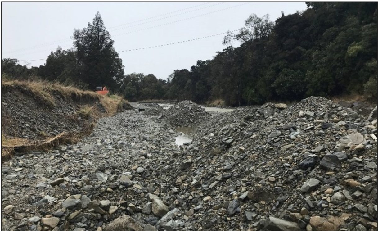
Figure 11-3: Looking towards the Ford at Blandswood from upstream (post July 2017 flooding)
