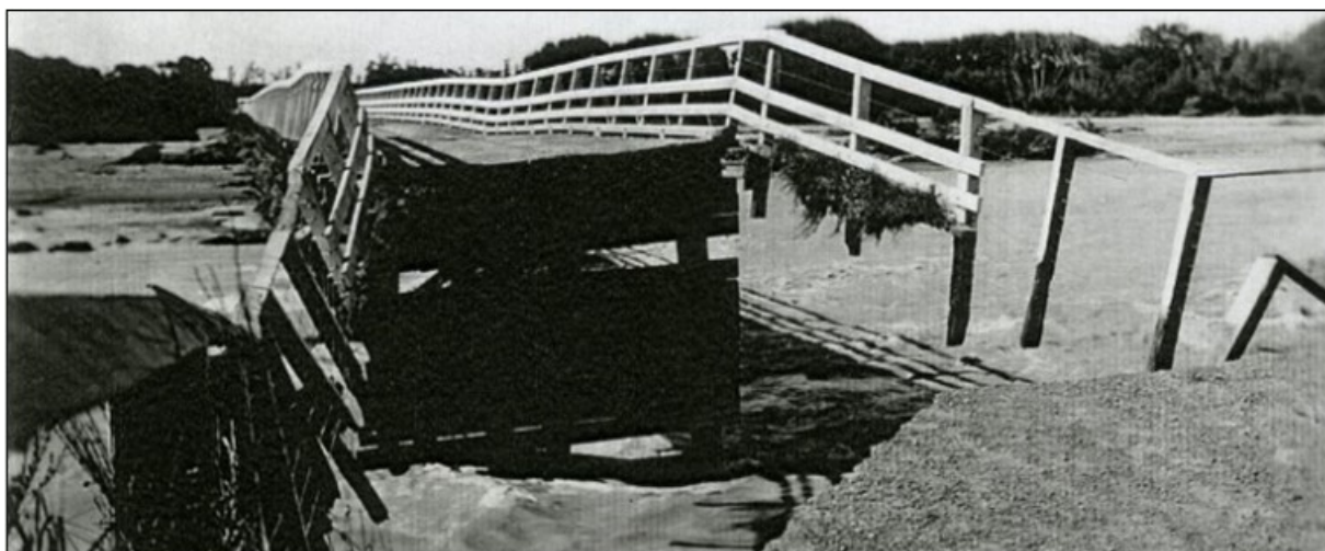
Figure 8-4: 18 April 1951 - Saleyards Bridge washout on south bank immediately downstream of the Stratheona hut settlement
