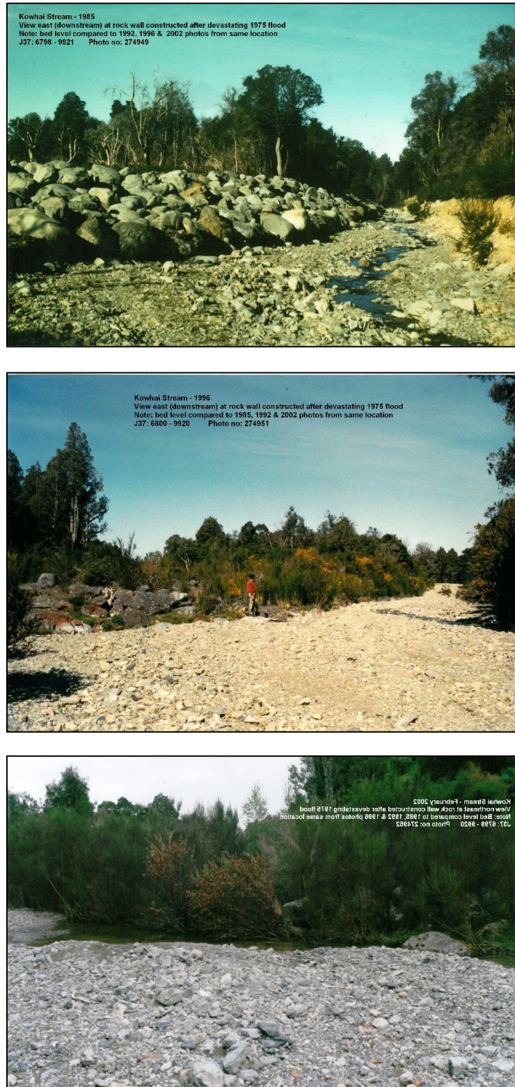
Figure 11-4: Series of photographs (Top: 1985, Middle: 1996 and Bottom: 2002) taken of rock protection put on true left stream bank upstream of ford following the devastating 1975 flood. Note photographs are all the same location and show the very rapid gravel bed aggradation occurring
