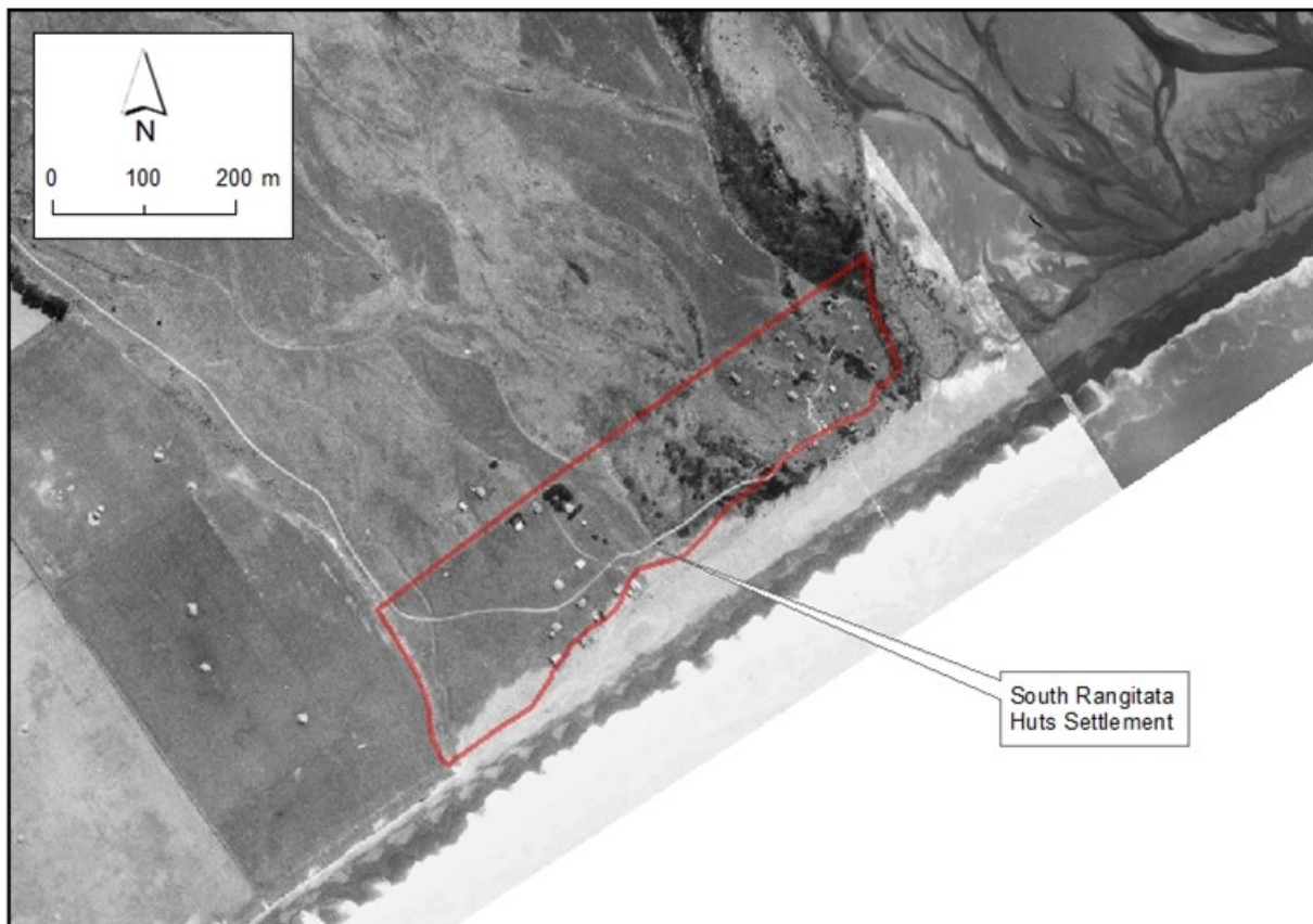
Figure 2-3: 1935-1939 aerial photograph showing South Rangitata hut settlement
