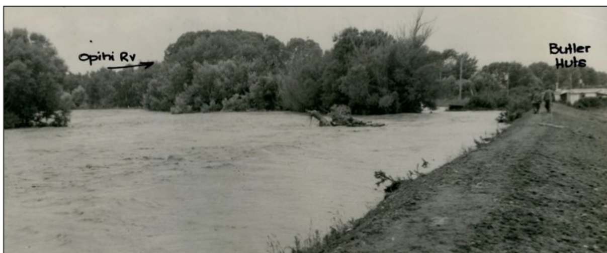
Figure 7-5: November 1952 - First Opihi River stopbank at Butlers Road hut settlement
