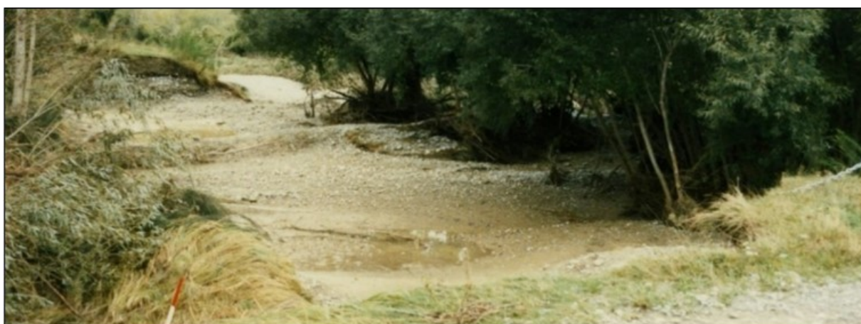
Figure 6-5: 13 March 1986 - breach through stopbank (40 m wide) looking from Mill Road downstream
