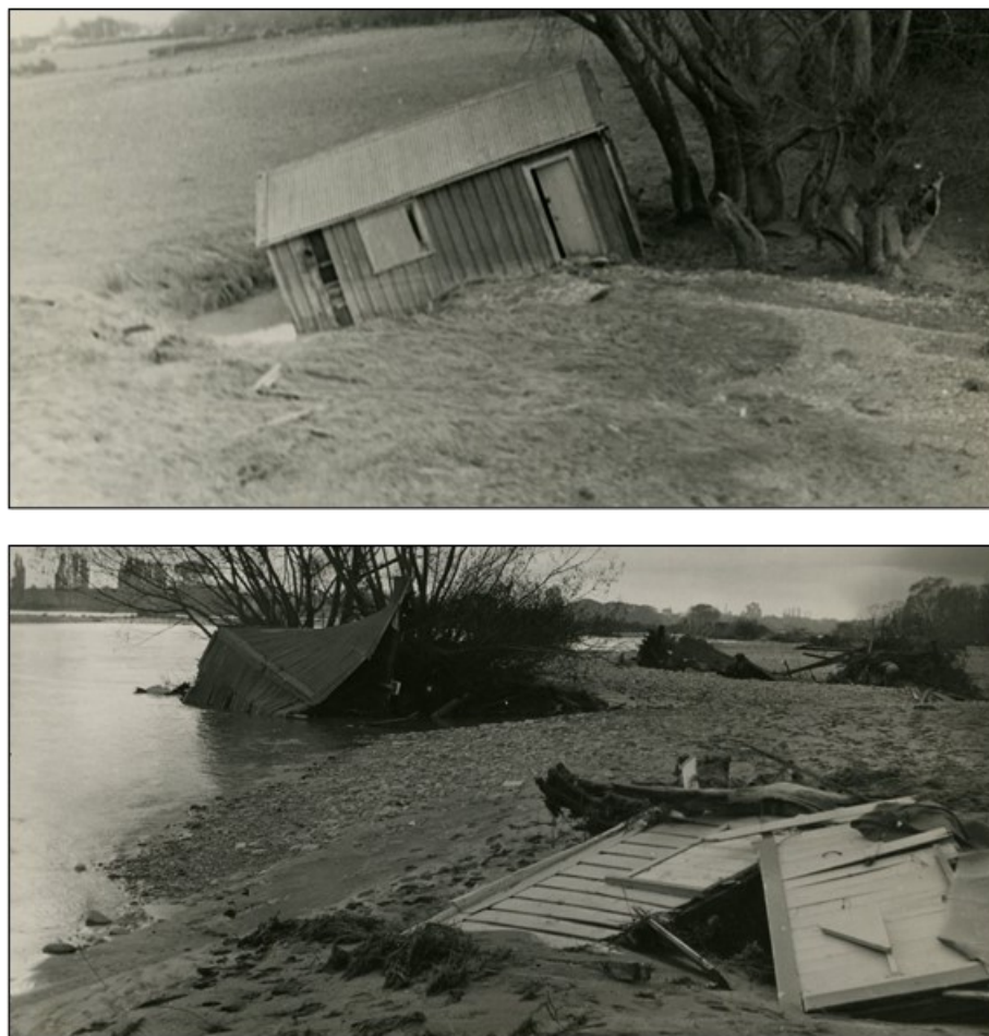
Figure 5-4: Aftermath of 18 April 1951 flood event in the Grassy Banks hut settlement area
