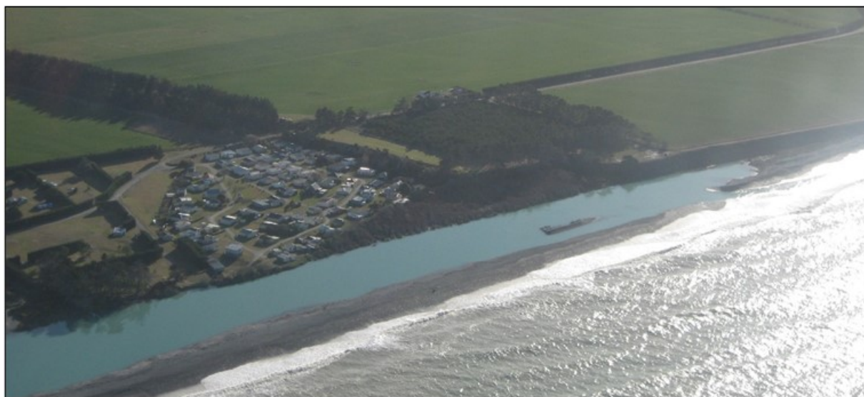
Figure 2-6: Rangitata River mouth on 26 June 2012. Mouth has migrated to north of the north bank huts which are visible in photograph. This was a few days after two huts were inundated at the South Rangitata hut settlement as a result of backwater flooding
