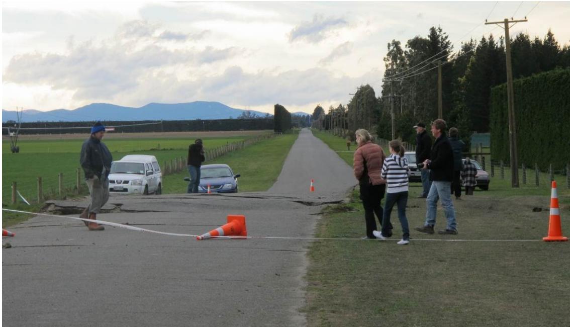
Figure 1.2 Surface fault rupture on the Greendale Fault at Highfield Road in Selwyn District (see Figure 1.1 for location) during the 4 September, 2010, Darfield (Canterbury) Earthquake. Before the earthquake, the road was straight and the ground was flat. At this location, surface fault rupture formed a ~40 m wide zone of fractures and broad folds in the ground resulting from mostly sideways ('strike-slip') ground shift of ~4.5 m. In addition, the south side (near the camera) was bulged up by about 1 m. Photo: D.J.A. Barrell, 5 September 2010.
