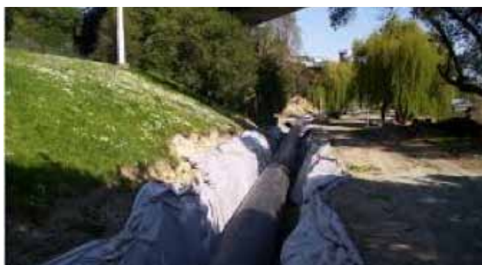
Three Waters Infrastructure
