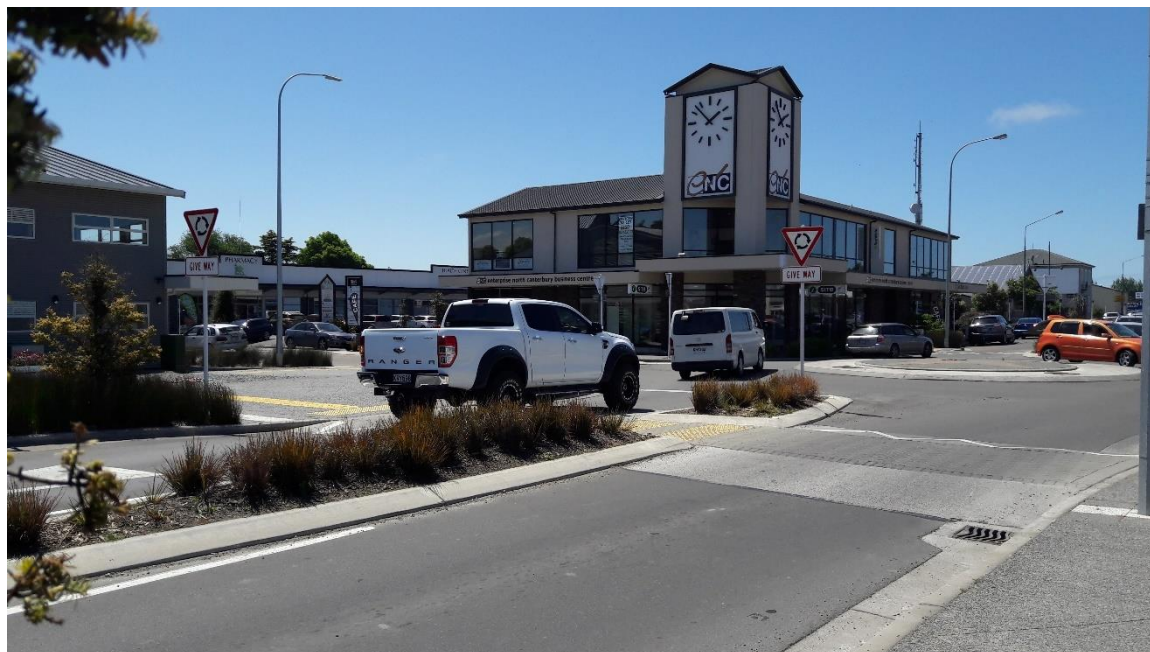
Figure 7 Raised platform on approach at an urban Roundabout
