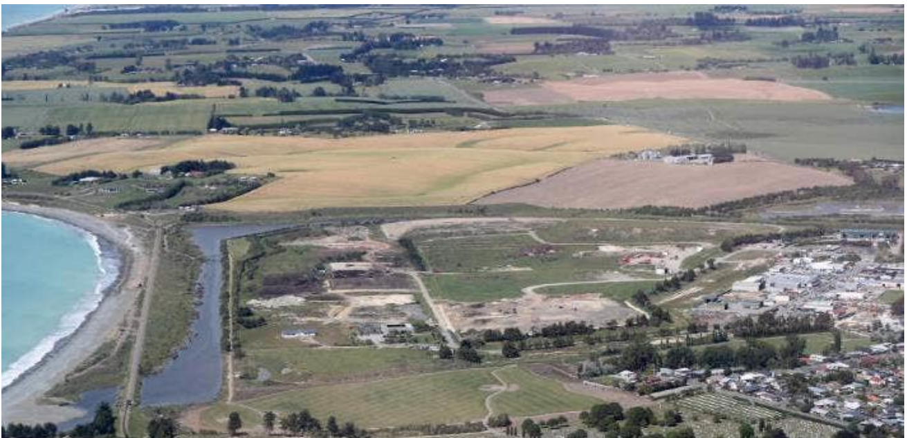
Figure 10 Image of the Redruth Facility
