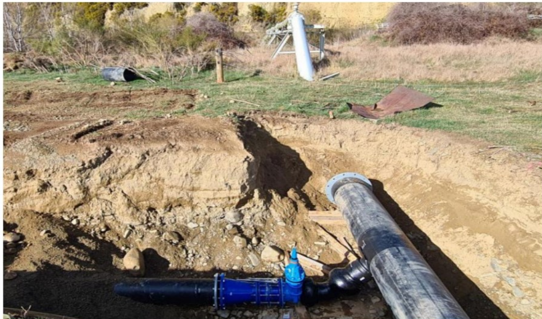
Contract 2468 – Pareora Pipeline Section 1
