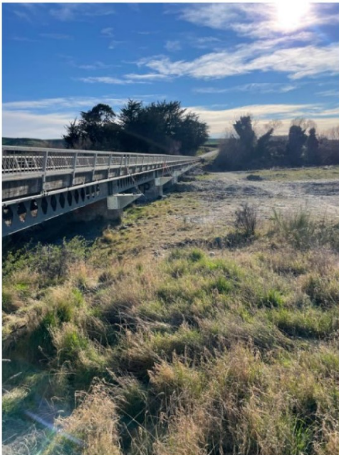
Holme Station Road bridge brackets have been installed ready for the beams and stainless steel pipe
