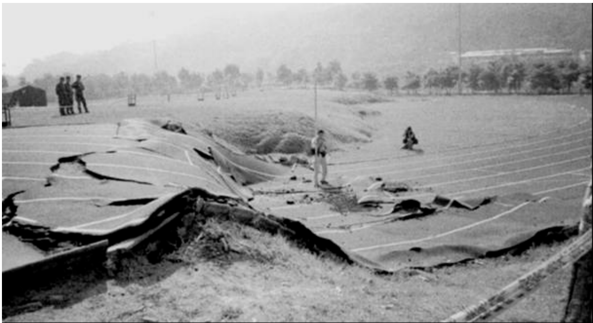
Figure 6.1 Fault scarp formed on the Chelungpu Fault during the magnitude 7.6 Chi-Chi Earthquake, Taiwan, 1999. The disrupted running track shows damage typical of a reverse fault ground-surface rupture, which is well expressed on the brittle surface (note the smoother rupture across grass behind). This location lies on a stream terrace that is younger than the previous rupture event on the fault, so that there was no scarp here before the earthquake. This example illustrates the sorts of effects that can be expected across fault scarps in the Timaru District the next time any particular fault experiences a surface rupture earthquake. Photo from Kelson et al. (2001).
