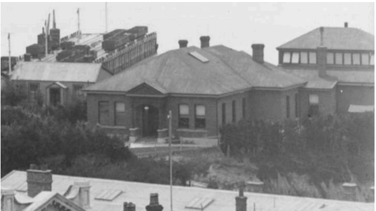
Detail of 1910 view of Timaru, with cottage on adjacent site to club, 1/1-08810-G, Alexander Turnbull Library, Wellington.
