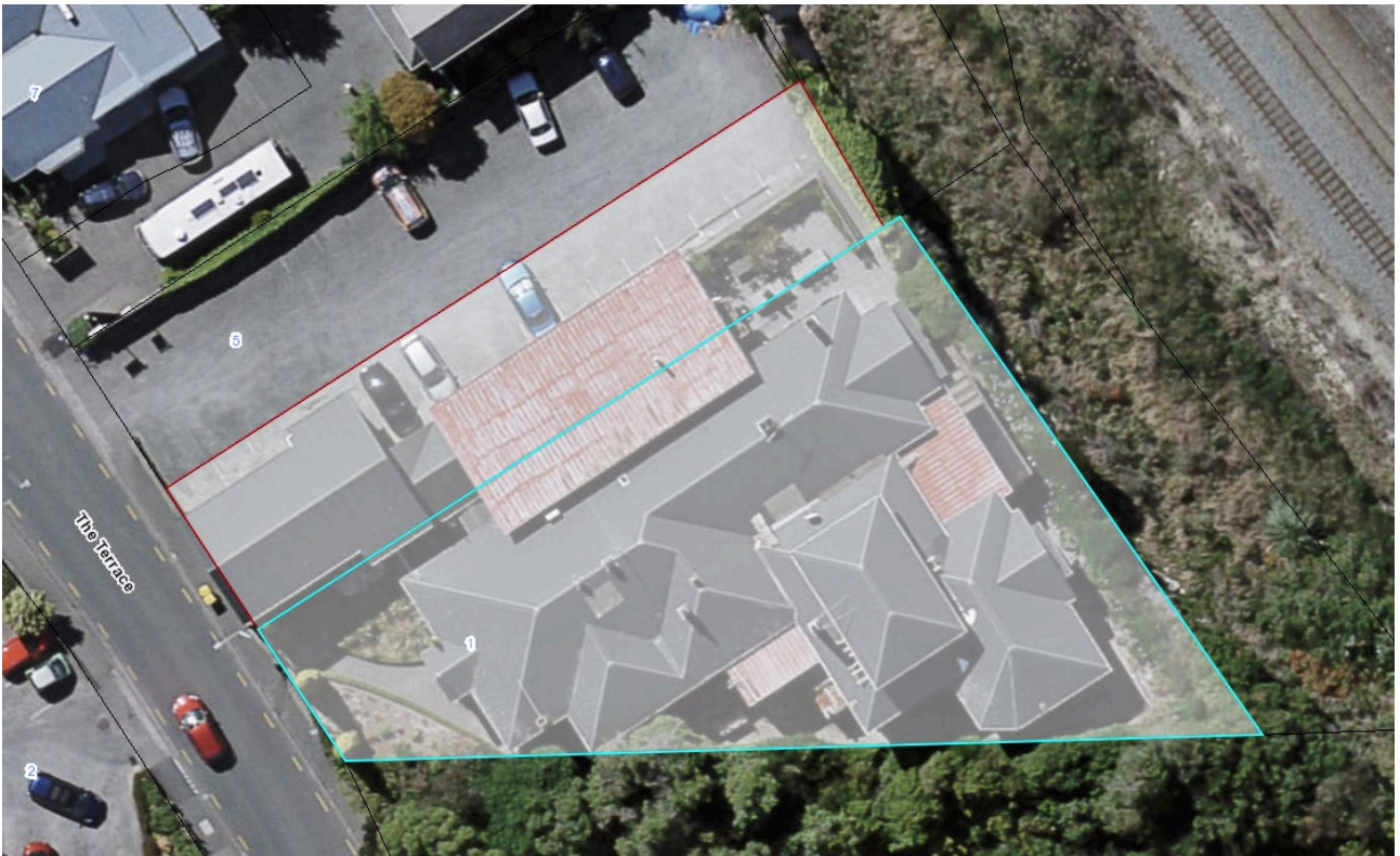
Extent of setting, including the squash court site on the northern boundary of the primary parcel, 1 The Terrace, Timaru.
