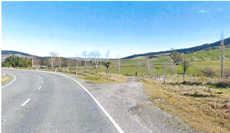
Figure 4: 1180 Geraldine - Fairlie Highway (State Highway 79) existing eastern access point.
