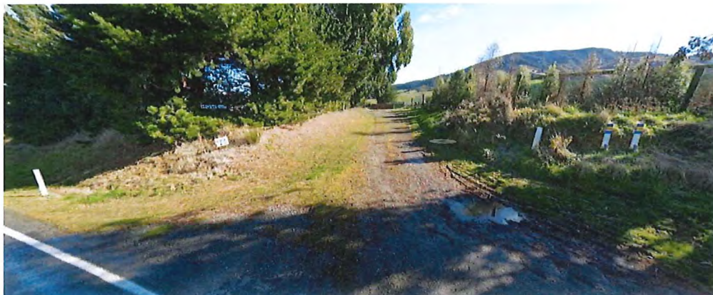
Figure 2: Geraldine - Fairlie Highway (State Highway 79) and Howe Road intersection.
