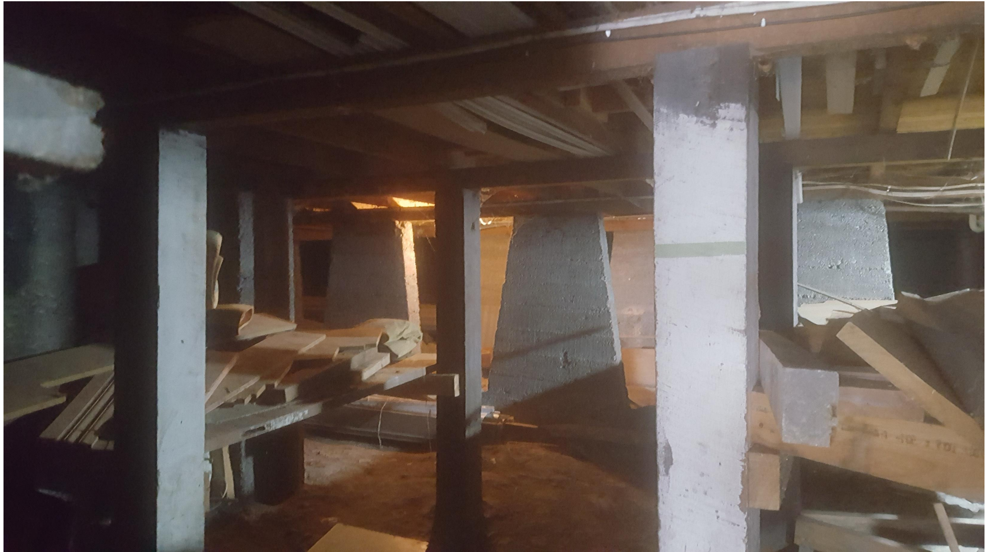
Foundations under the west wing, showing the tapered shape.
