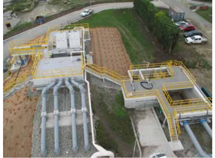
Aerial view of Domestic screening structure and peak flow pump station
