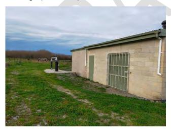
The reservoir at Tripp Street Reserve holds 2,275m³, approximately 12 hours storage at average peak demand. Pressure reduction occurs when the draw off from the reservoir is high and exceeds inflow. The reservoir underwent a structural assessment in 2017 which deemed it to have an effective remaining life of 10 years and vulnerable to seismic events within the vicinity.
