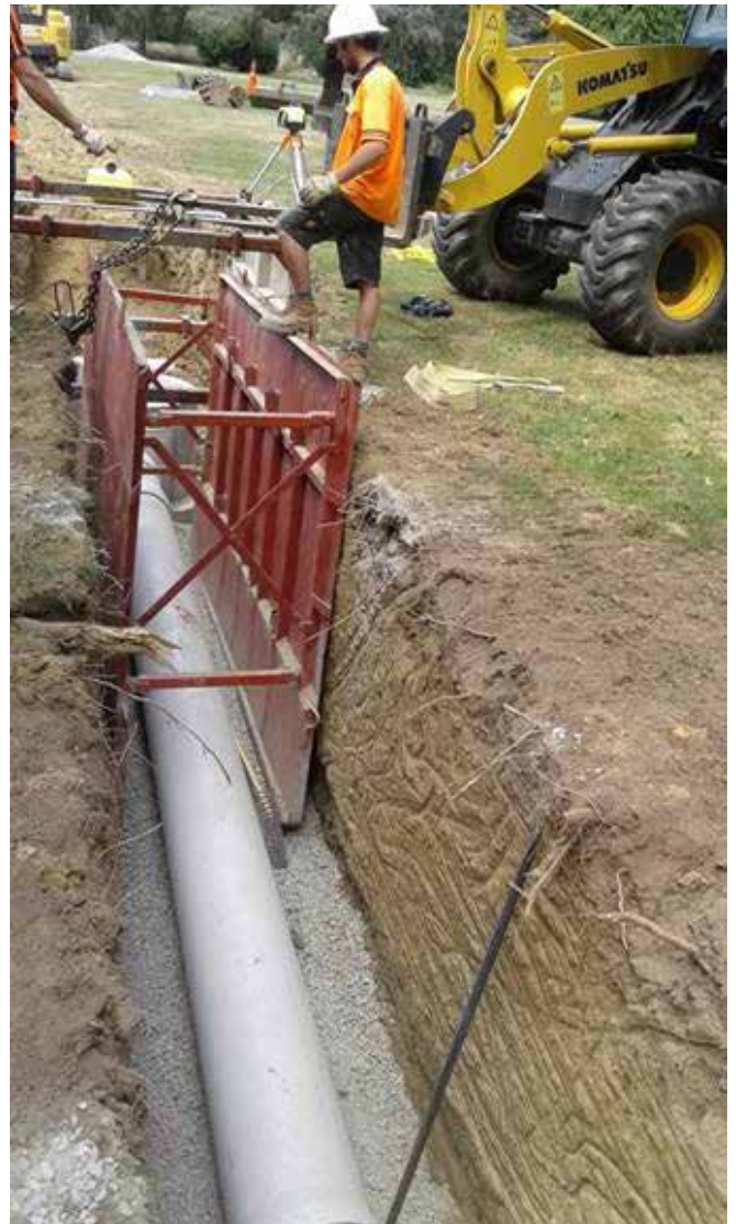
Domain Avenue Sewer main Renewal
