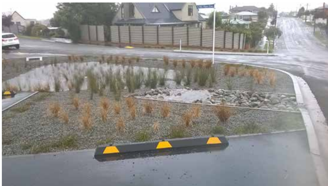
Kauri Street raingarden
