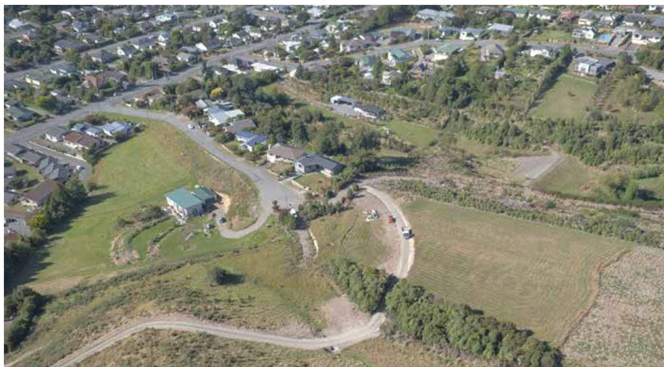
Drone image of new Geraldine shared walking cycling track
