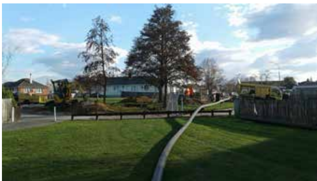
Dunkirk Street Sewer main Rehabilitation
