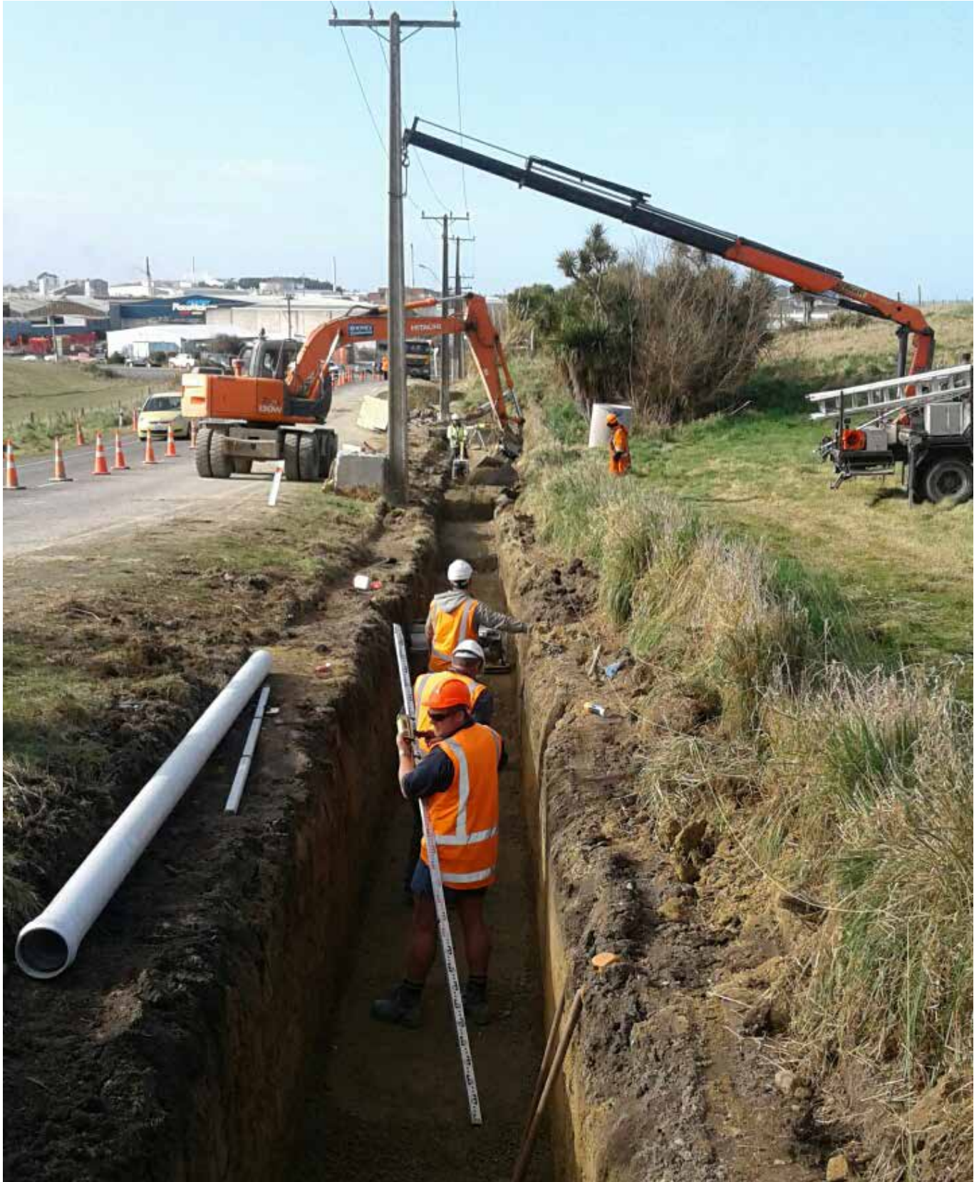
Blair Street Sewer main Renewal
