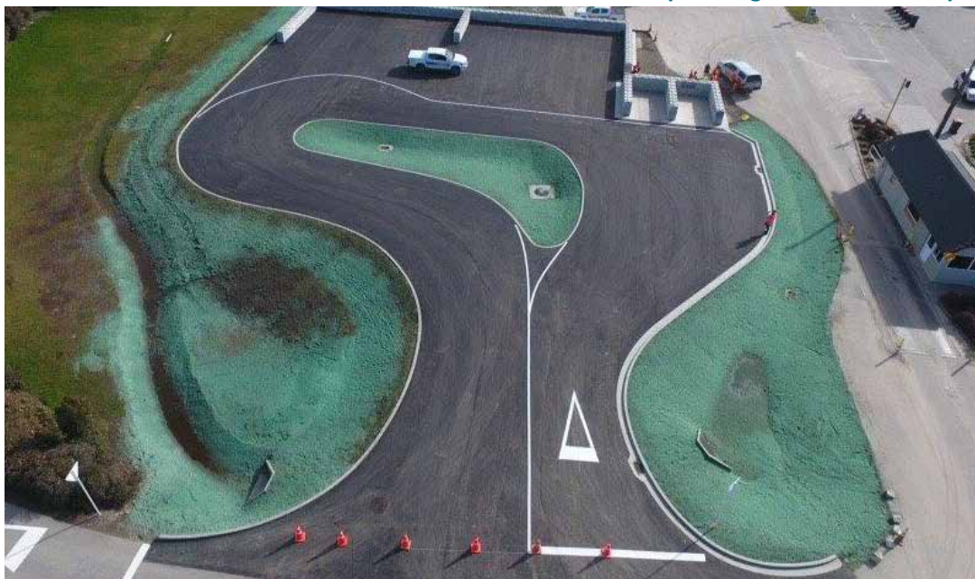
Greenwaste Drop-off site Construction at Redruth Resource Centre
