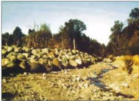
Figure 5: View of site on completion of protection works (1985)
