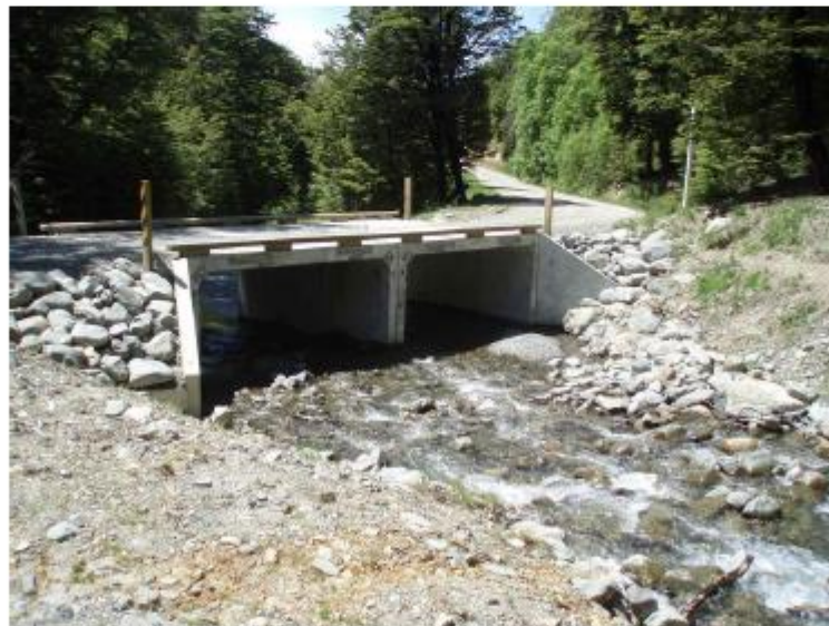
Figure 9: Example of Multicell Box Culvert
