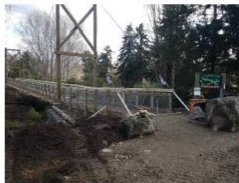
Figure 18: Recently Constructed pedestrian suspension bridge (Centennial Park)
