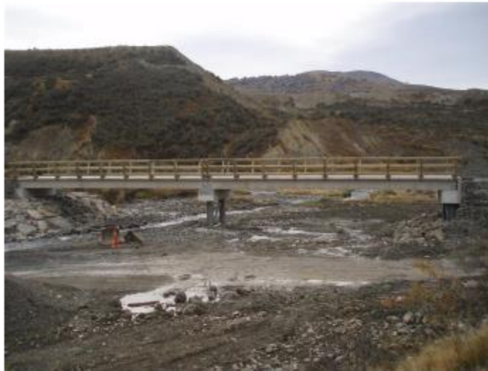
Figure 12: Example of Single Lane Vehicle Bridge
