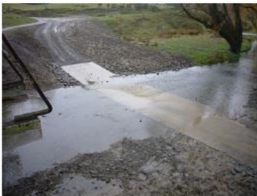
Figure 13: An example ford following final construction
