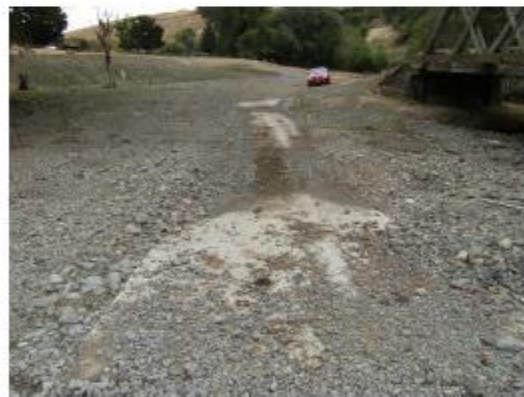
Figure 14: View of same ford approximately 6 months after construction, showing gravels accumulating on running surface
