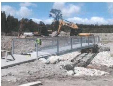
Figure 17: Example of lightweight steel superstructure (single span shown)
