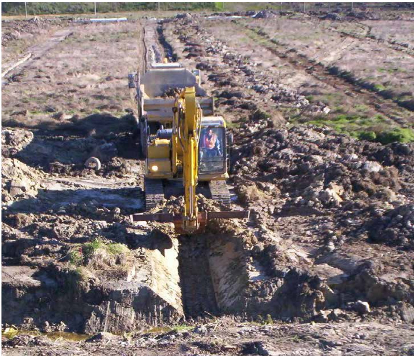
New cell foundations for Redruth Landfill
