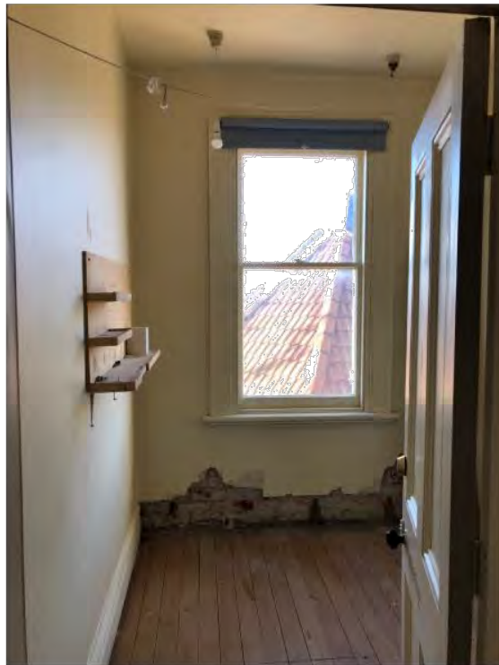
Figure 31 Space 22, servants bedroom
