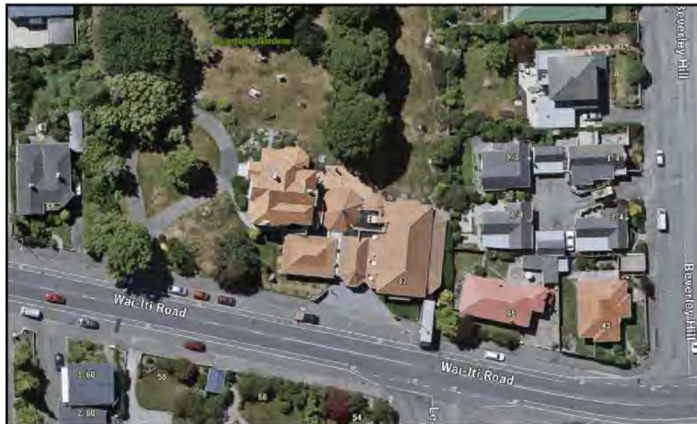
Figure 1: Aerial image of the Aigantighe Art Gallery (centre of image) in relation to Wai-iti Road, Timaru.
