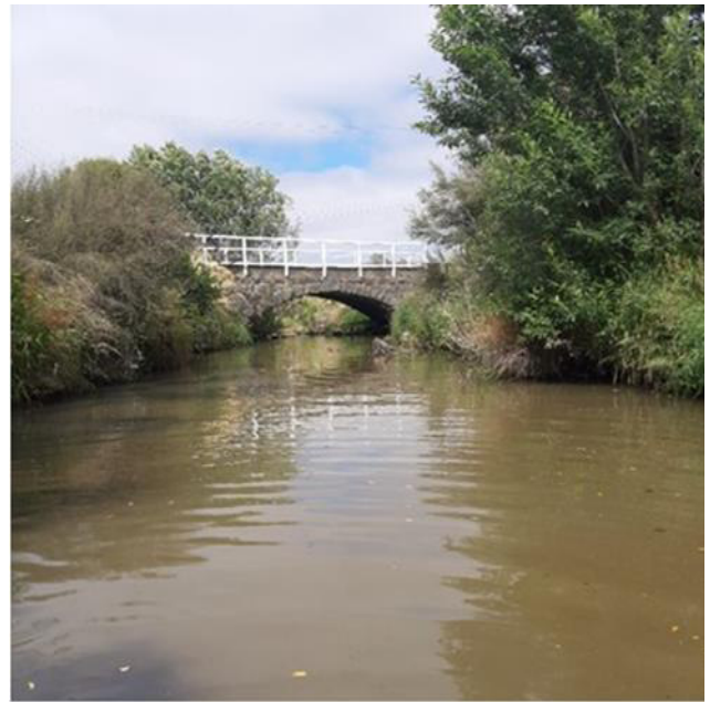
Figure 4-11: Downstream reach of Ōtipua - Saltwater Creek
