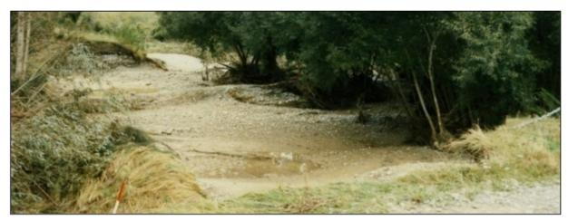
Figure 6-5: 13 March 1986 - breach through stopbank (40 m wide) looking from Mill Road downstream
