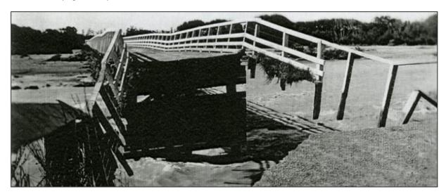
Figure 8-4: 18 April 1951 - Saleyards Bridge washout on south bank immediately downstream of the Stratheona hut settlement
