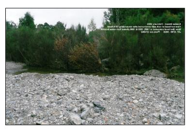
Figure 11-4: Series of photographs (Top: 1985, Middle: 1996 and Bottom: 2002) taken of rock protection put on true left stream bank upstream of ford following the devastating 1975 flood. Note photographs are all the same location and show the very rapid gravel bed aggradation occurring
