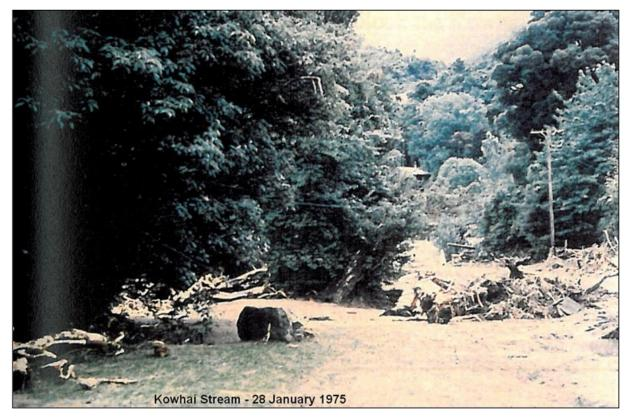
Figure 11-5: Lookout Road, Blandswood following 1975 flood event [Source: Hall (1993), plate 4]. Note large boulder thrown onto road in centre bottom of shot and huge volume of debris on road
