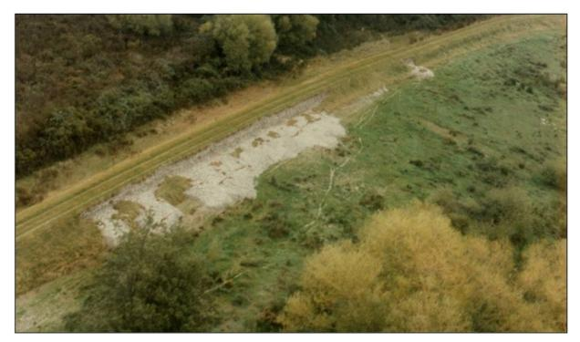
Figure 9-5: Opihi River stopbank on true right bank ~300 m upstream of Collett Road following overtopping during the 13 March 1986 flood
