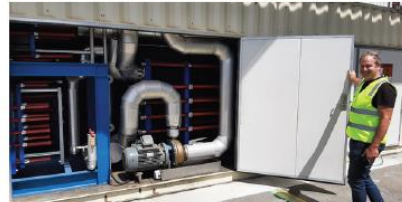
Adrian Peltason shows part of the Brewery refrigeration system, using ammonia as refrigerant in an outdoor located unit. The chill is transferred by heat exchanger to less-hazardous glycol for speed circulation through the plant.
