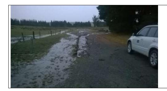
Clark Road Culvert – indicative of culvert problems to remedy on the network.
