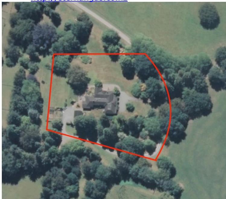
Extent of setting, limited to homestead's garden setting, 965 Cleland Road, Totara Valley.
