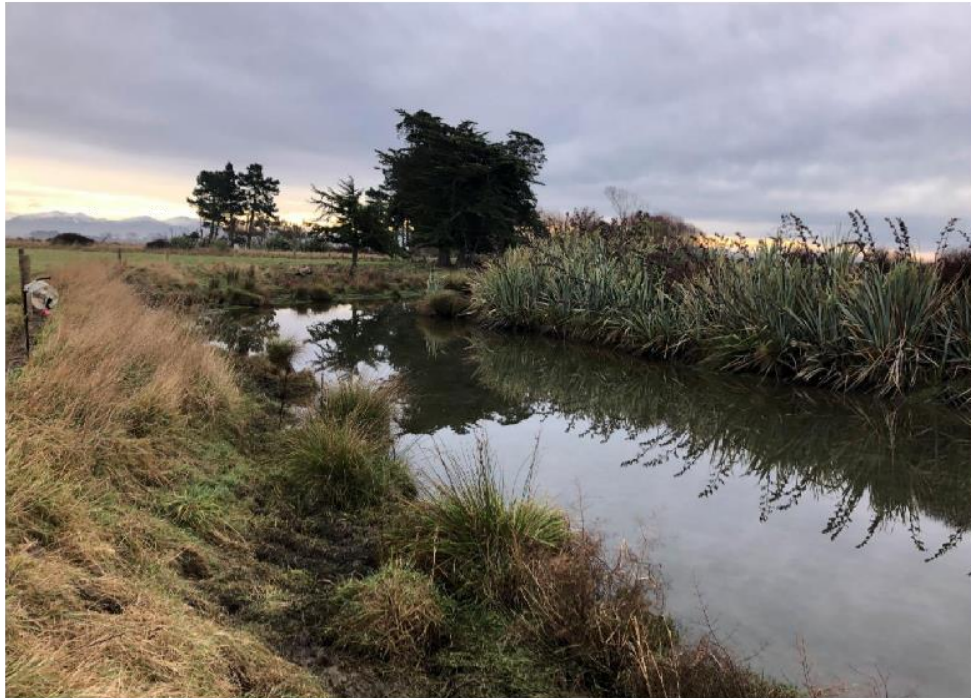
Looking towards Prattley road, far bank fenced and near bank to be done.
