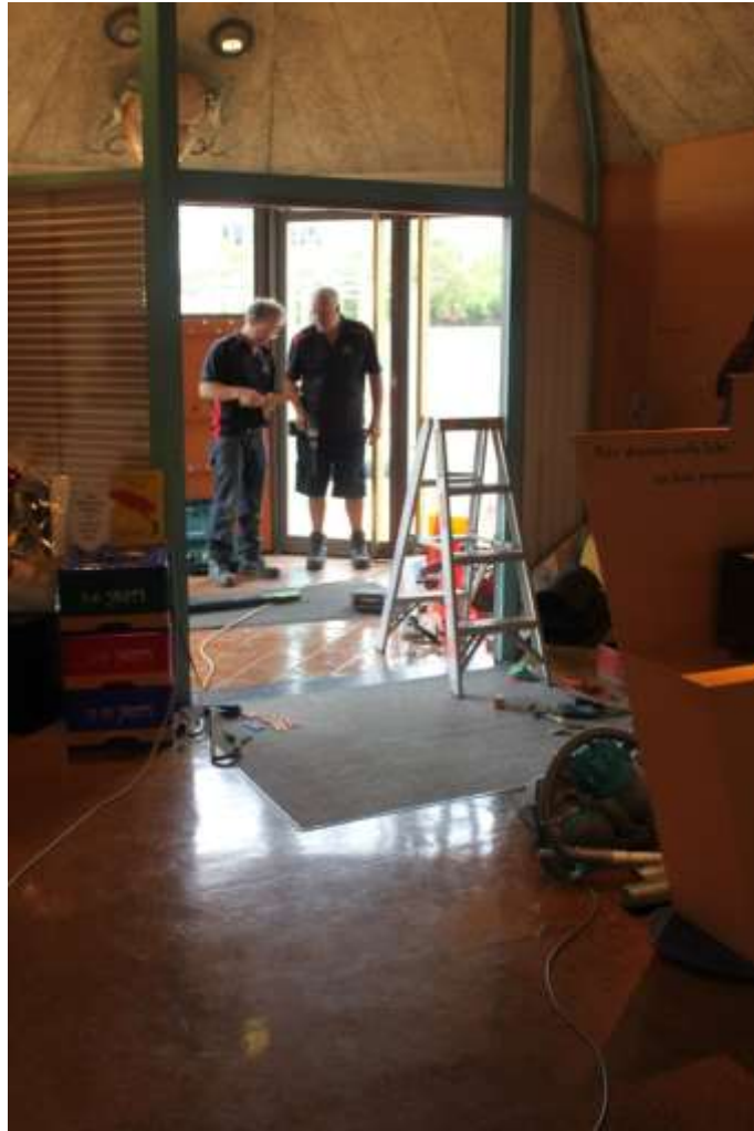
Installation of the new gallery entrance doors November 2013
