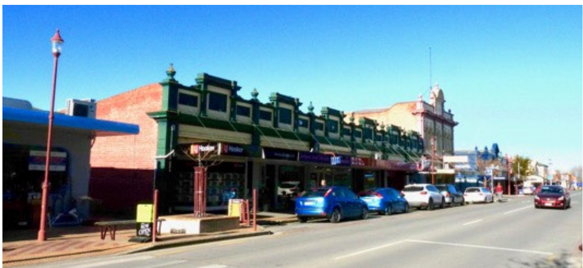
View south with the former Job Brown's Beehive Stores (heritage item # 117, 1901-2) to the right of centre.
